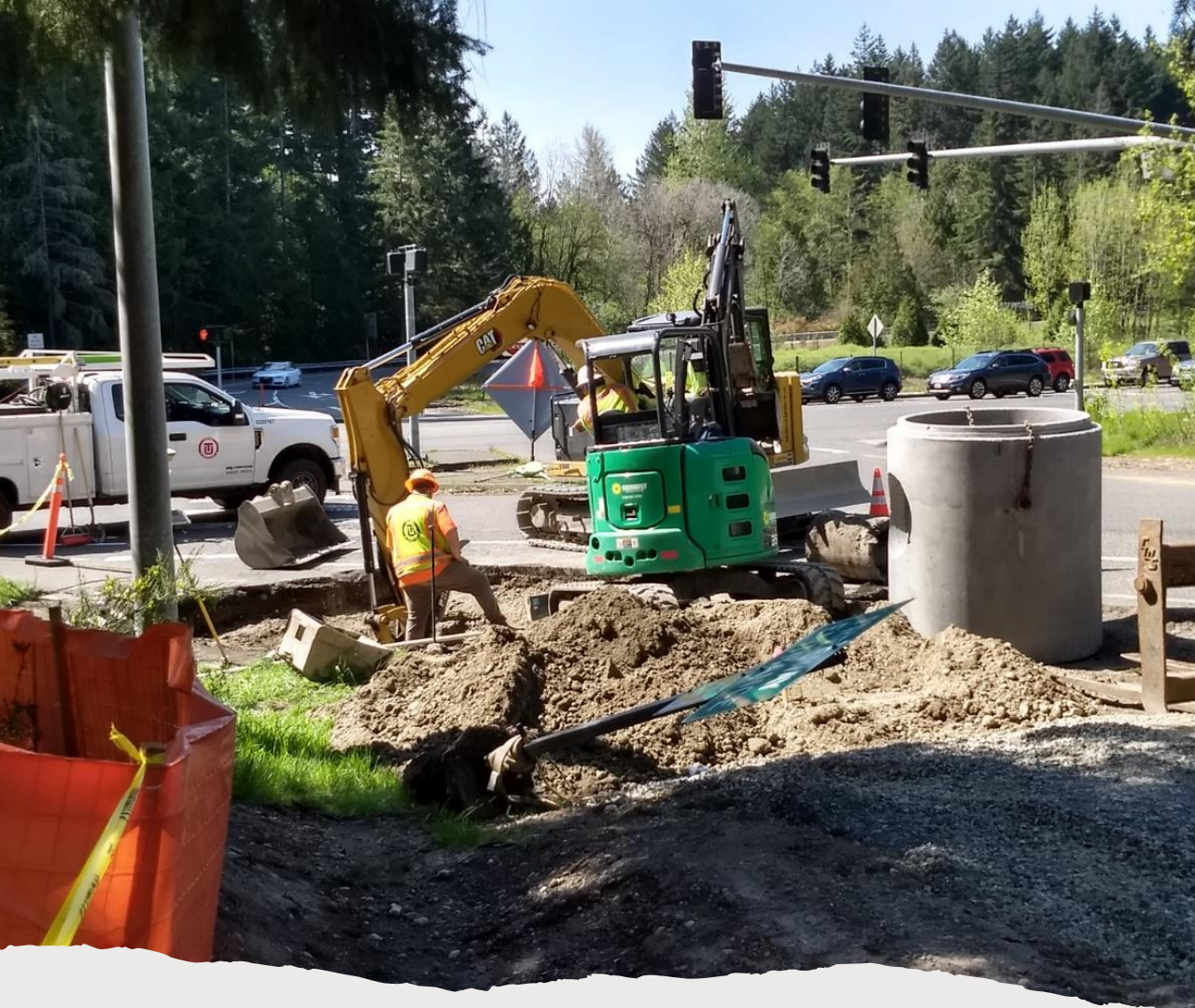
May 3 - CB installation on Ramp Utility Rough in on Ped Connection to Flyer Stop
