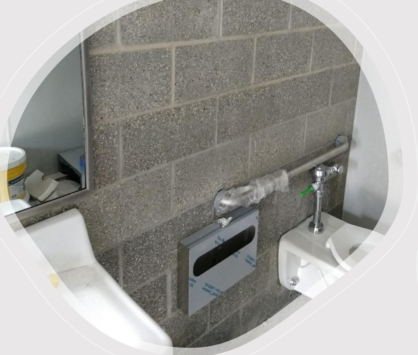
Inside Finishing Restroom and Mechanical Room
