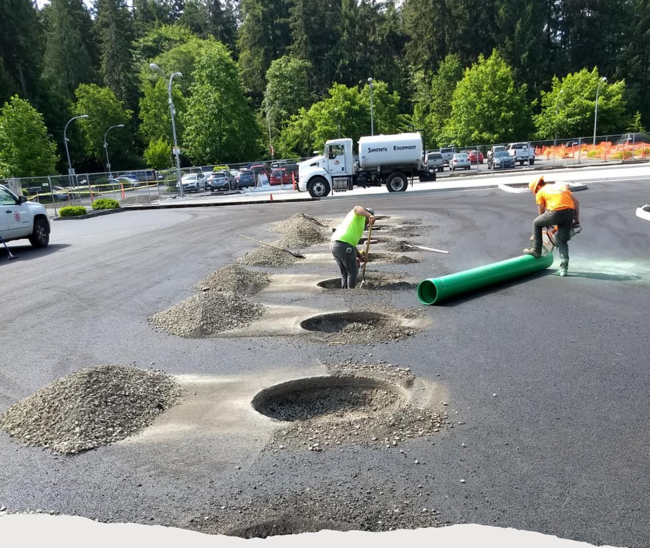
North Lot – Stormwater Facility Replacing Collars in repaired area
