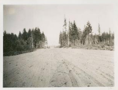
3:30 P.M. August 23, 1934 Looking ahead from Station 119+00. Finished grade. # 28
