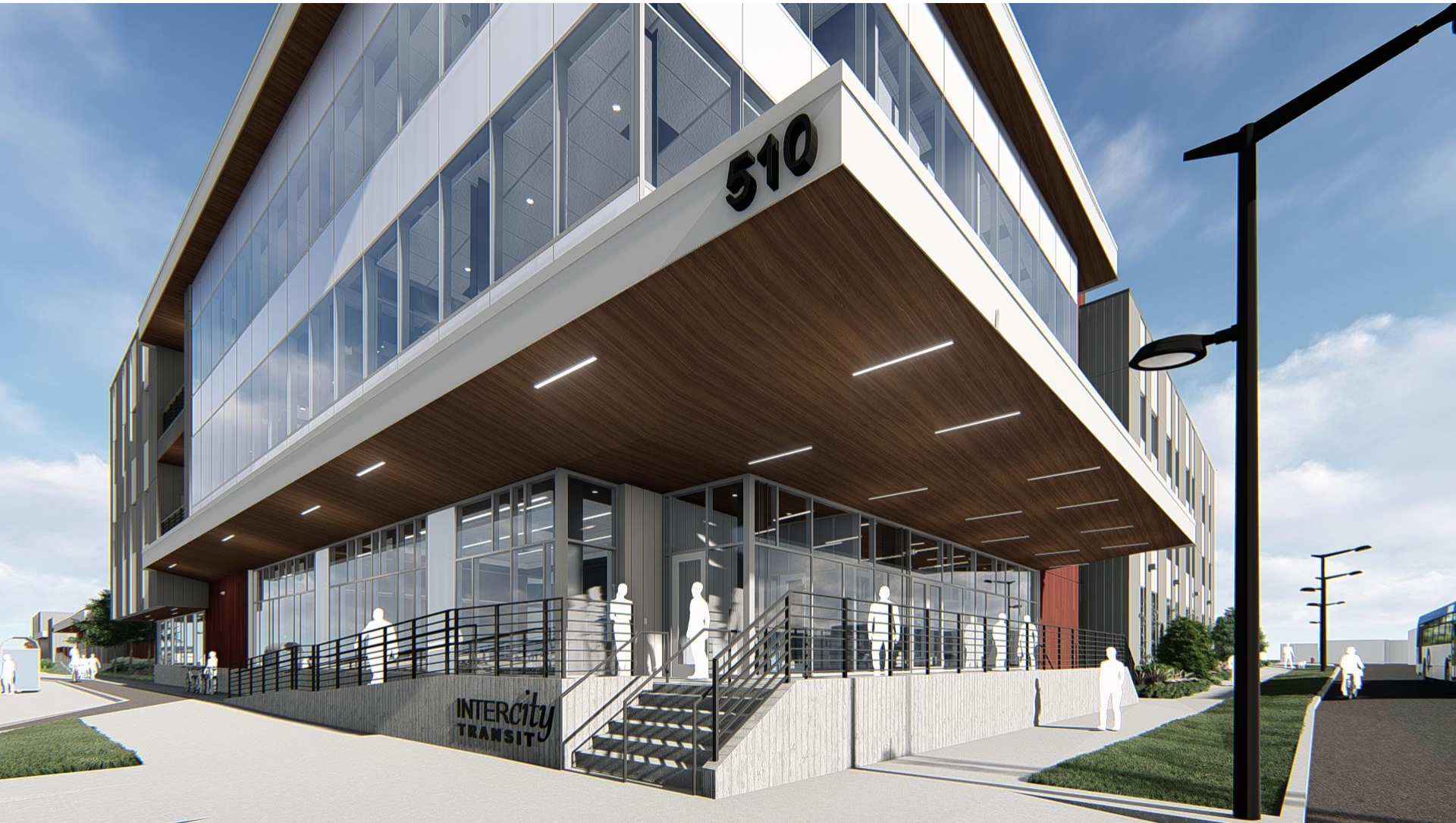
ENTRY PORCH * LOBBY
