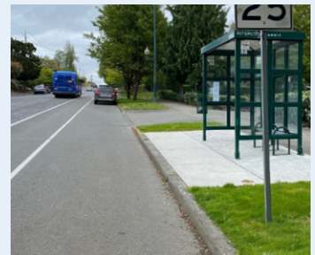
Wide shoulder stop on 4th Ave. at Central St., eastbound
