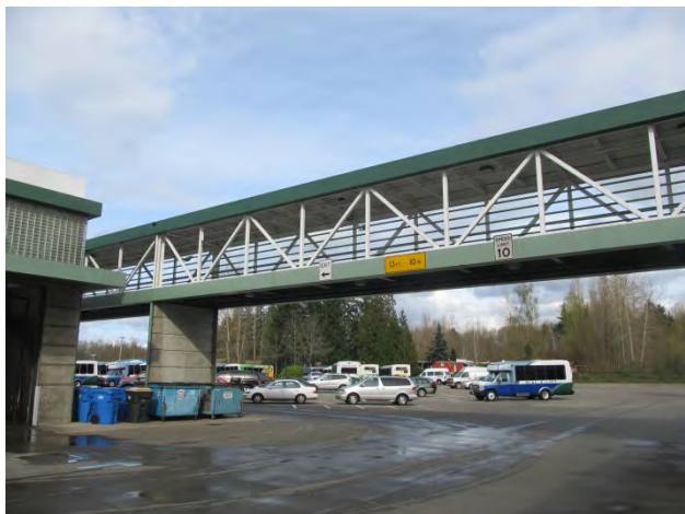
Photo 3 shows a general view of the east bridge.
