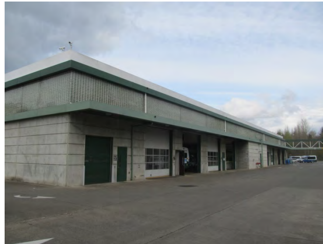
Photo 2 shows a general view of the south façade of the maintenance facility.
