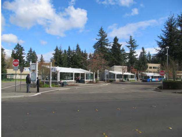
Photo 30 shows a general view of the Lacey Transit Center.
