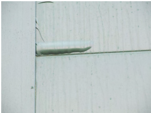
Photo 11 shows an example of the rusting that is occurring along the joint between the fascia and glass block windows.
