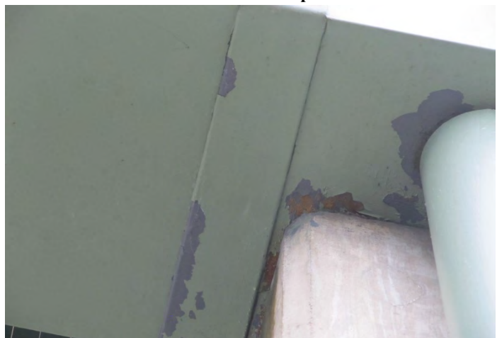
Photo 17 shows a general view of the bridge surfaces. The inset photo shows an example of the rust that was observed at the base of one of the posts.
