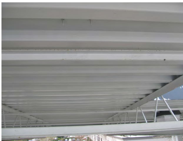
Photo 5 shows the results of an adhesion test conducted on the siding at the east end of the building. Adhesion was poor (ASTM D6677: 0).
