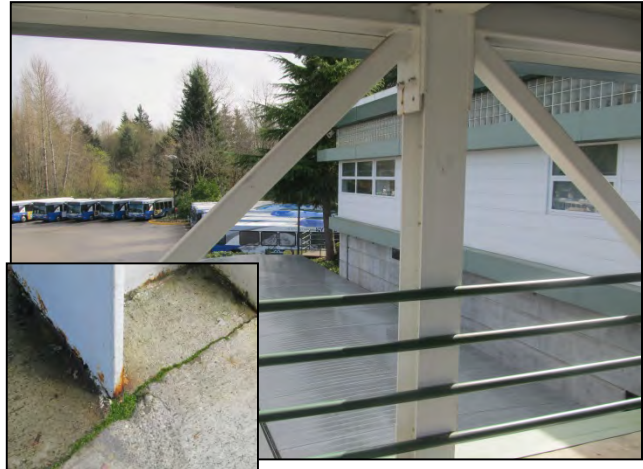
Photo 17 shows a general view of the bridge surfaces. The inset photo shows an example of the rust that was observed at the base of one of the posts.
