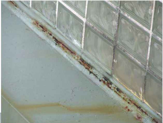
Photo 11 shows an example of the rusting that is occurring along the joint between the fascia and glass block windows.
