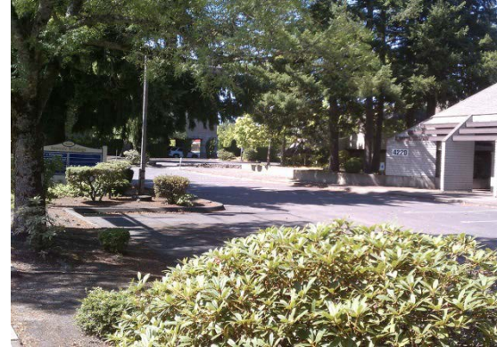
Main Building from 6th Ave SE (Existing)
